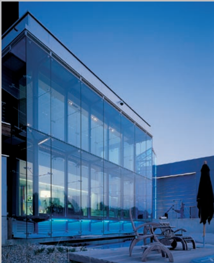
Living Tomorrow Public Building, Brussels, Belgium
