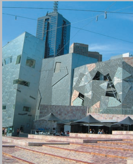
Conference Square Commercial Building Sydney, Australia
